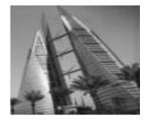
turbines at a perpendicular angle and increases air speed as much as 30 percent in each of the 95 ft wide turbine rotors. The turbines supply about 15 percent of the electricity used by the skyscraper
